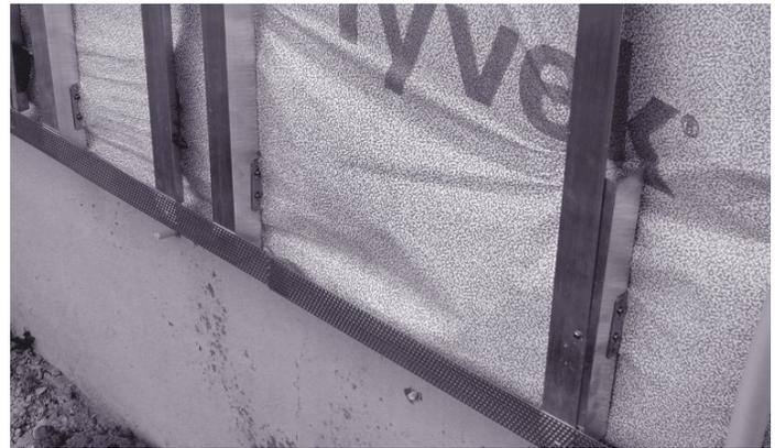
**Diagram of the installation of the galvanised and aluminium profiles for board widths >1,875 mm**
