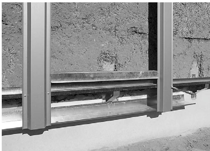
When using the DEKMETAL load-bearing construction, the same principles apply to the spacing of vertical profiles and anchoring elements – see the table of the Maximum axial distances of anchoring elements in chapters 7.1.3.1 Application of the CETRIS® VARIO boards and 7.1.3.2 Application of CETRIS® PLANK boards.
